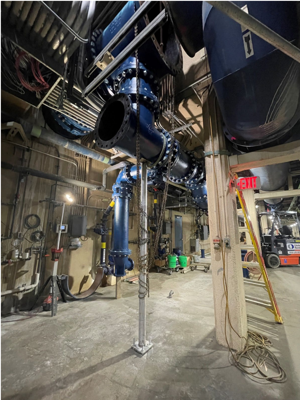
Photo of new north-side pump supply header being installed.
