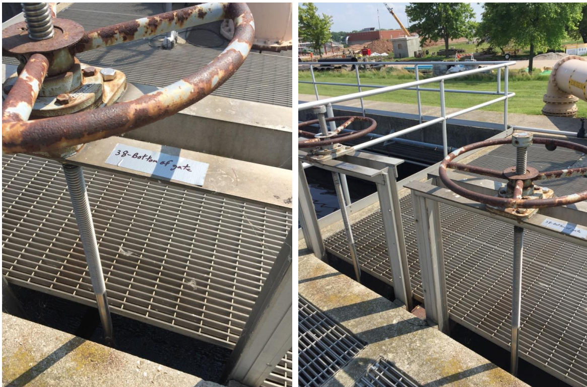
38. Gate between Splitter Box T-20 and Channel 1 (at Aeration Basins) – Bottom of gate (survey only)
