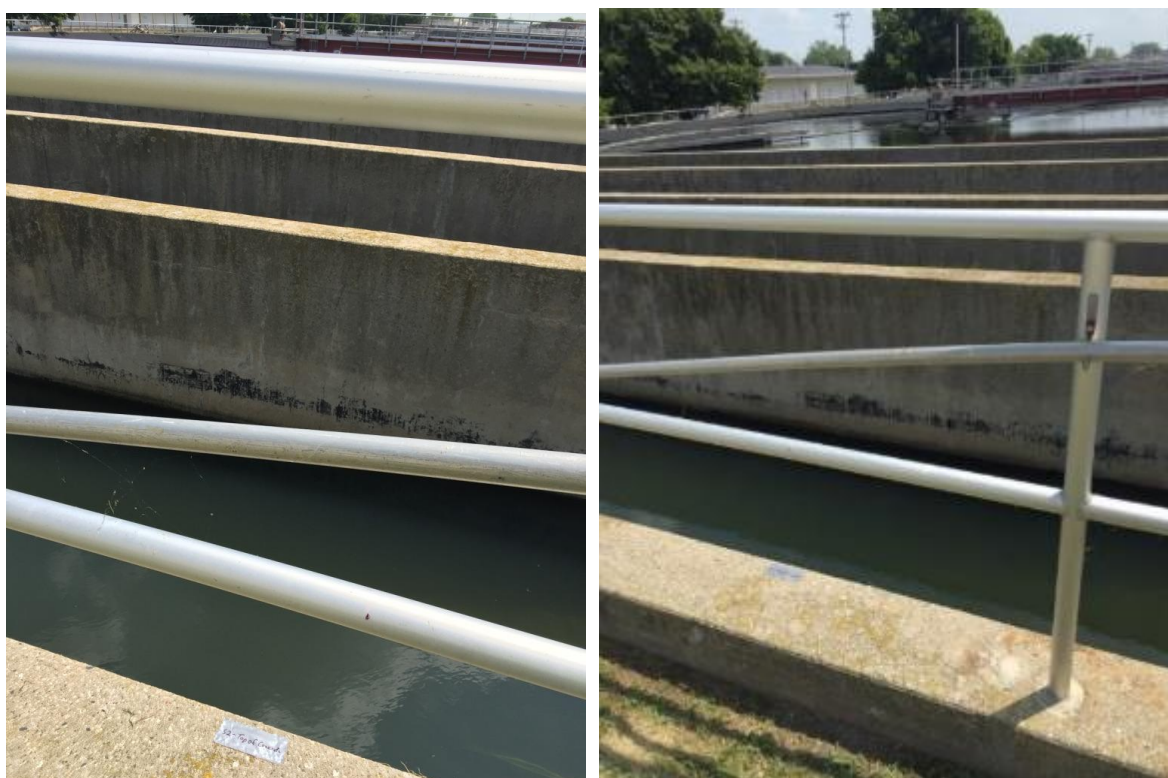
52. Upstream of Chlorine Contact Basin No. 1 Parshall Flume – Top of concrete
