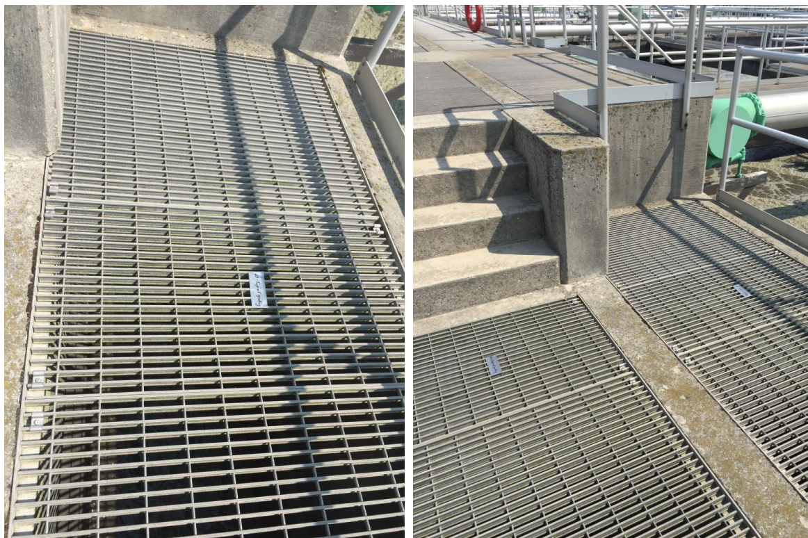
27. South Aeration Basin effluent channel – Top of grating
