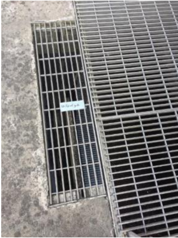
50. Filter bypass overflow (west) – Top of gate (survey only)
