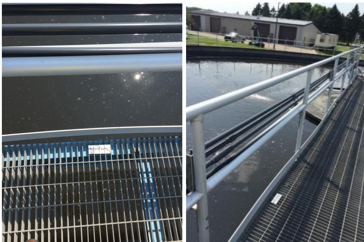
28. North Intermediate Clarifier bridge – Top of grating
