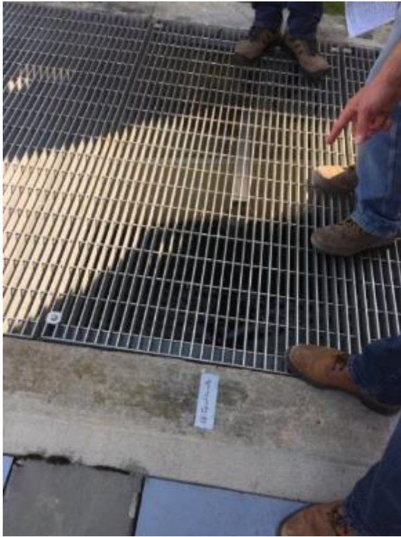
58. Final Effluent Flume – Top of concrete (survey only)
