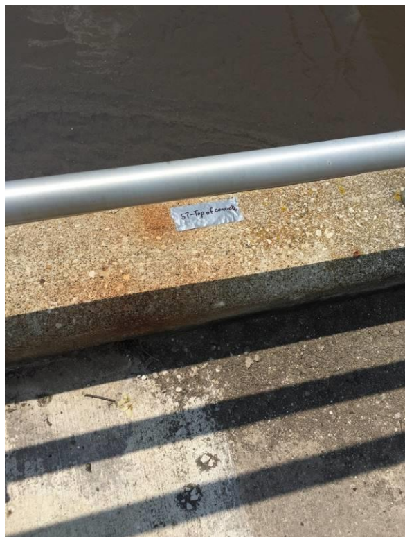
57. Upstream end of Aeration Basin No. 2 – Top of concrete
