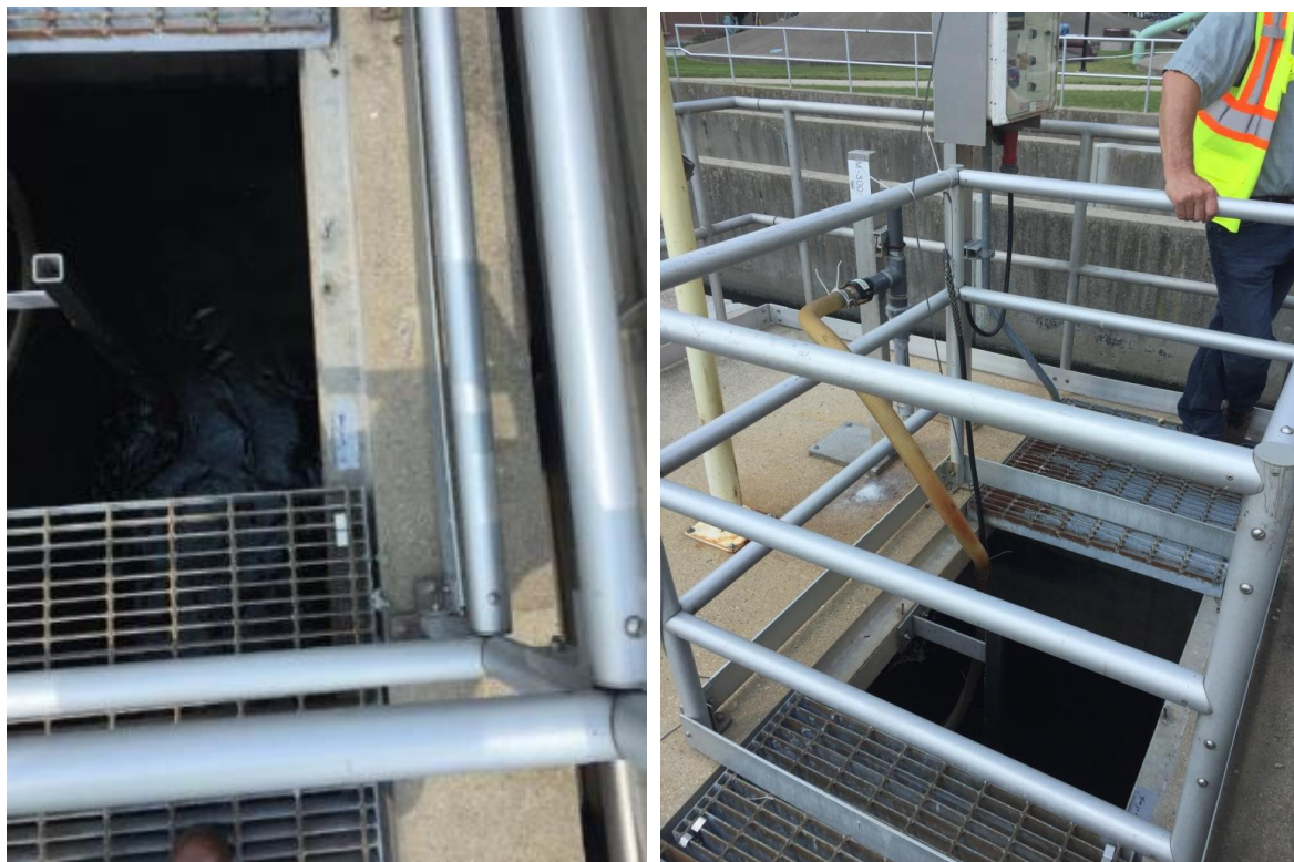
51. Just upstream of gate to Chlorine Contact Basin No. 2 – Top of angle
