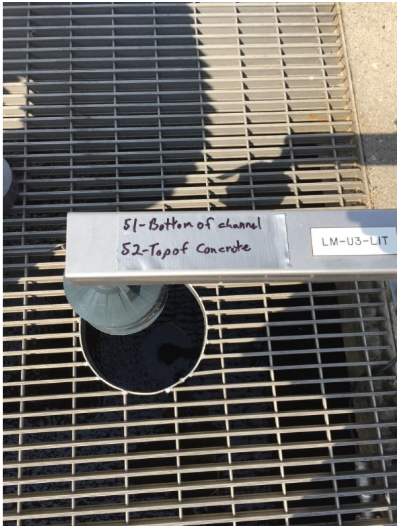
52. T-51 – Top of concrete
