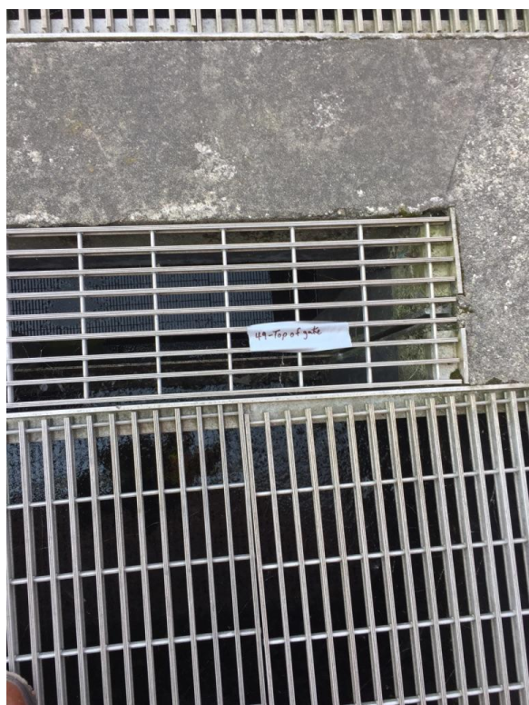
49. Filter bypass overflow (east) – Top of gate (survey only)
