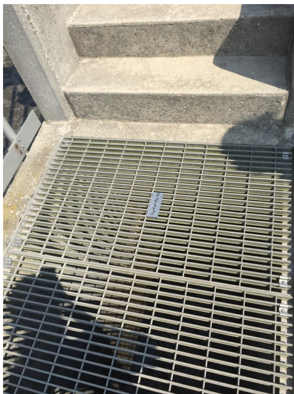
26. North Aeration Basin effluent channel – Top of grating (see 27 for additional photo)
