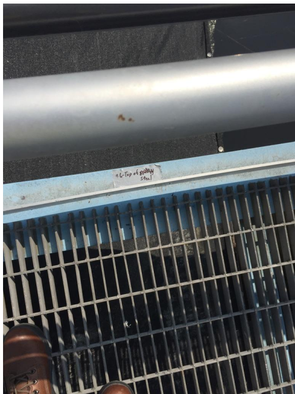
46. Southwest Final Clarifier launder (from bridge) – Top of steel
