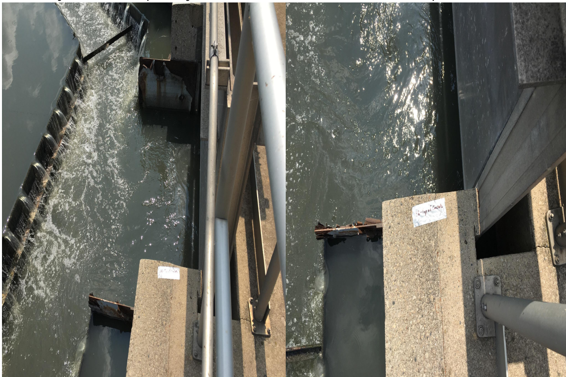
56. At Primary Basin No. 3 – primary effluent diversion box to GBF South – Top of concrete
