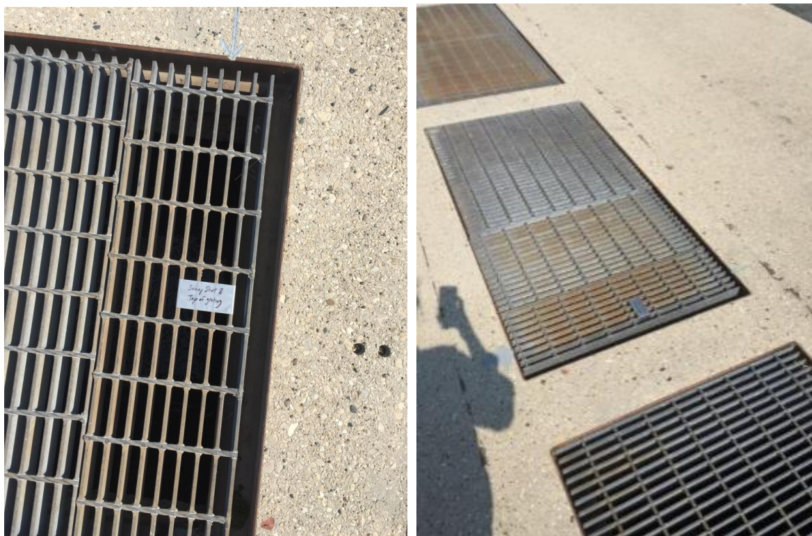
8. Parshall Flume downstream of screens (south) – Top of grating
