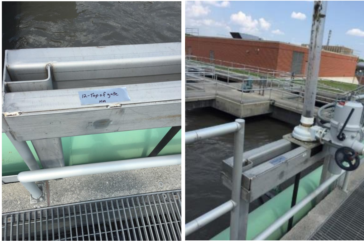
12. North Anoxic Basin gate (2 nd gate from the east) – Top of gate (survey only)
