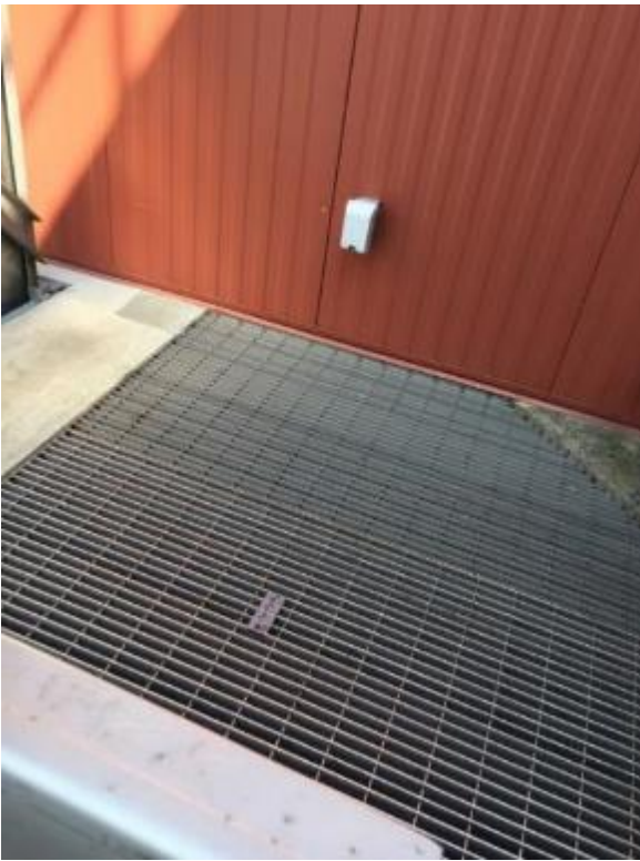
55. Channel on west side of UV Disinfection Building as shown – Top of grating
