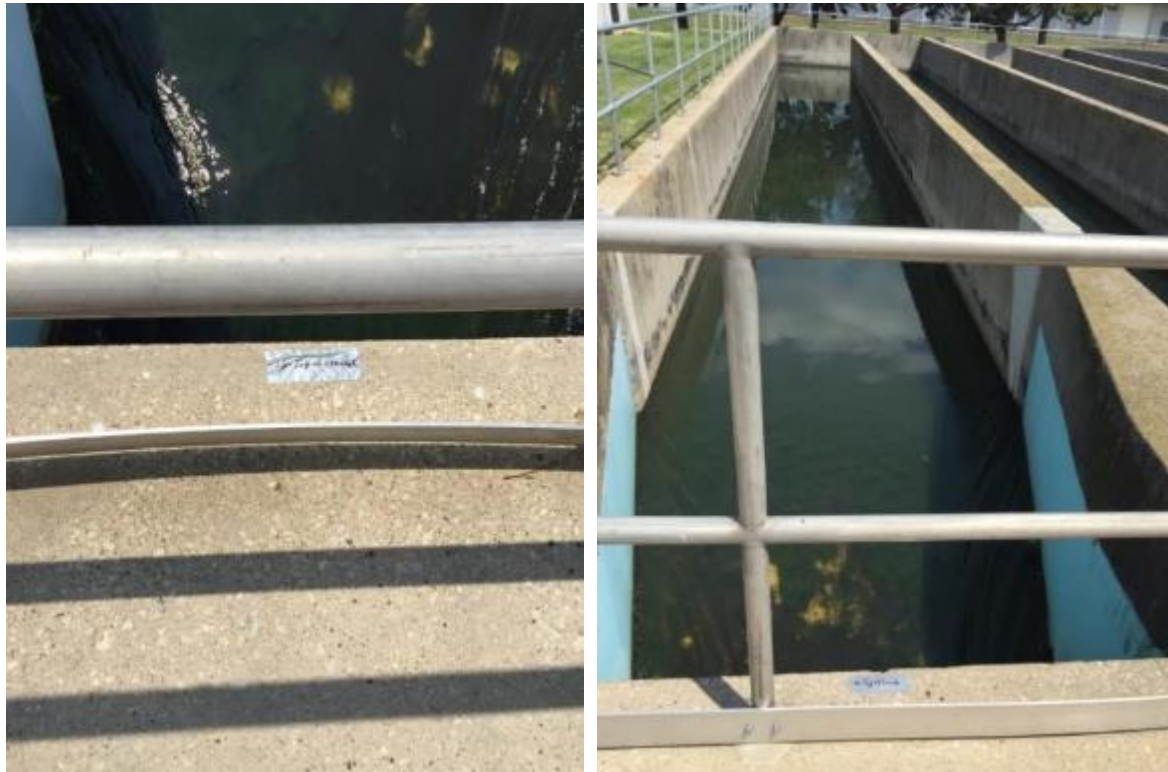
55. At bridge over Chlorine Contact Basin No. 2 Parshall Flume – Top of concrete
