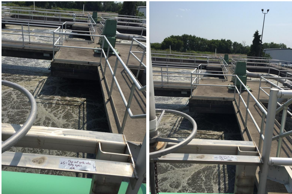
25. South Aeration Basin influent gate (west-most gate) – Top of gate when fully open (survey only)
