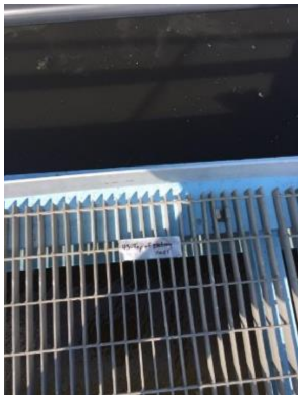
43. Southwest Final Clarifier bridge – Top of steel
