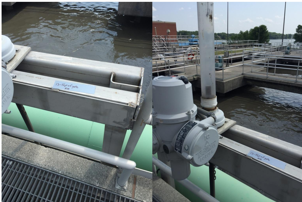
13. South Anoxic Basin gate (2 nd gate from the east) – Top of gate (survey only)
