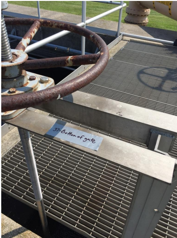
37. Gate at upstream end of Channel 2 (at Aeration Basins) – Bottom of gate (see 38 for additional photo) (survey only)
