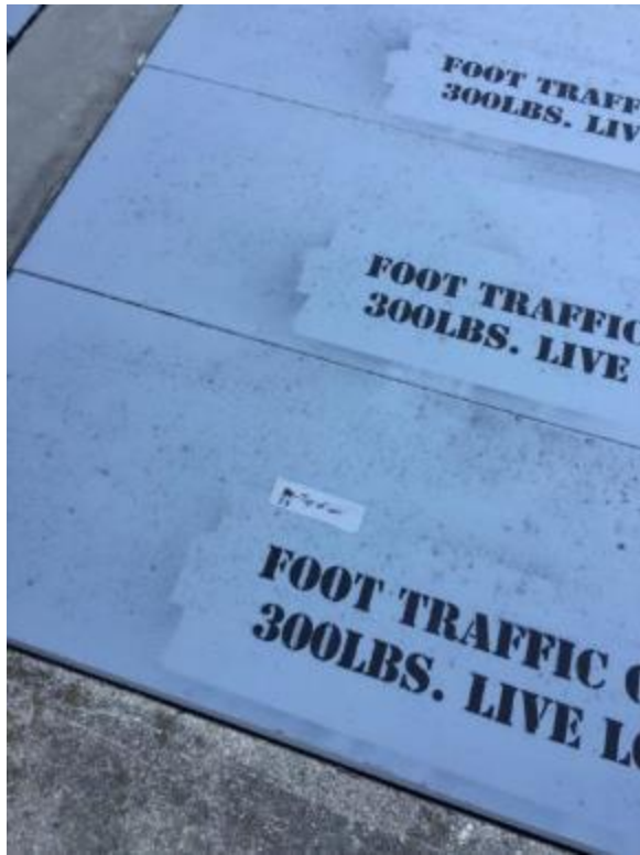
53. North channel downstream of UV – Top of weir (underneath grating) (survey only)
