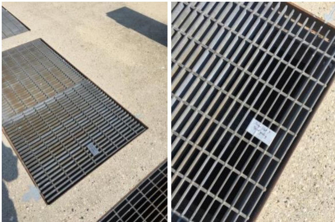
7. Parshall Flume downstream of screens (north) – Top of grating
