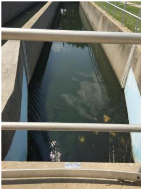
53. At bridge over Chlorine Contact Basin No. 1 Parshall Flume – Top of concrete
