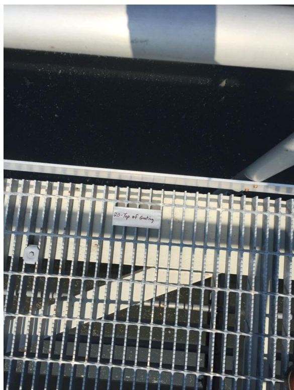
20. Primary Basin No. 3 bridge – Top of grating
