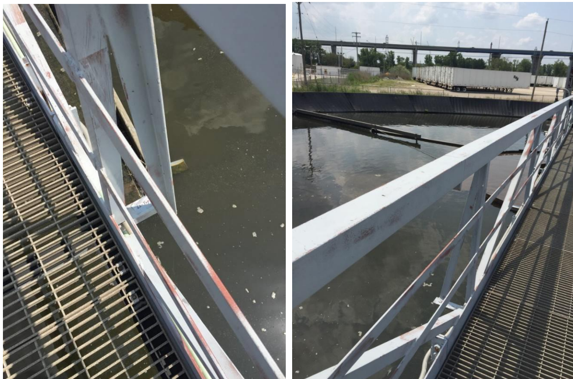
62. Secondary Clarifier No. 2 bridge – Top of support
