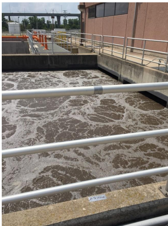
58. Downstream end of Aeration Basin No. 2 – Top of concrete
