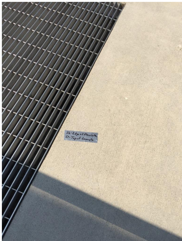
57. Final Effluent Flume – Top of concrete
