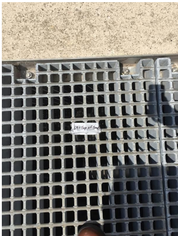
59. Channel just south of Mechanical Building – Top of grating
