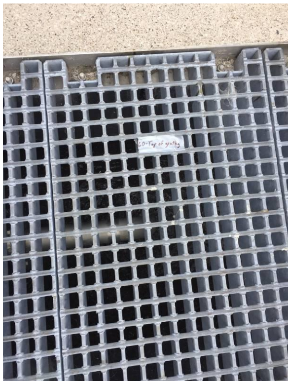
60. Channel just north of Electrical Building – Top of grating
