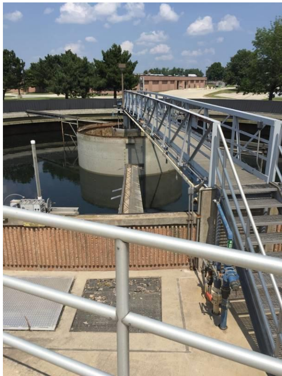
61. Secondary Clarifier No. 1 bridge – Top of support
