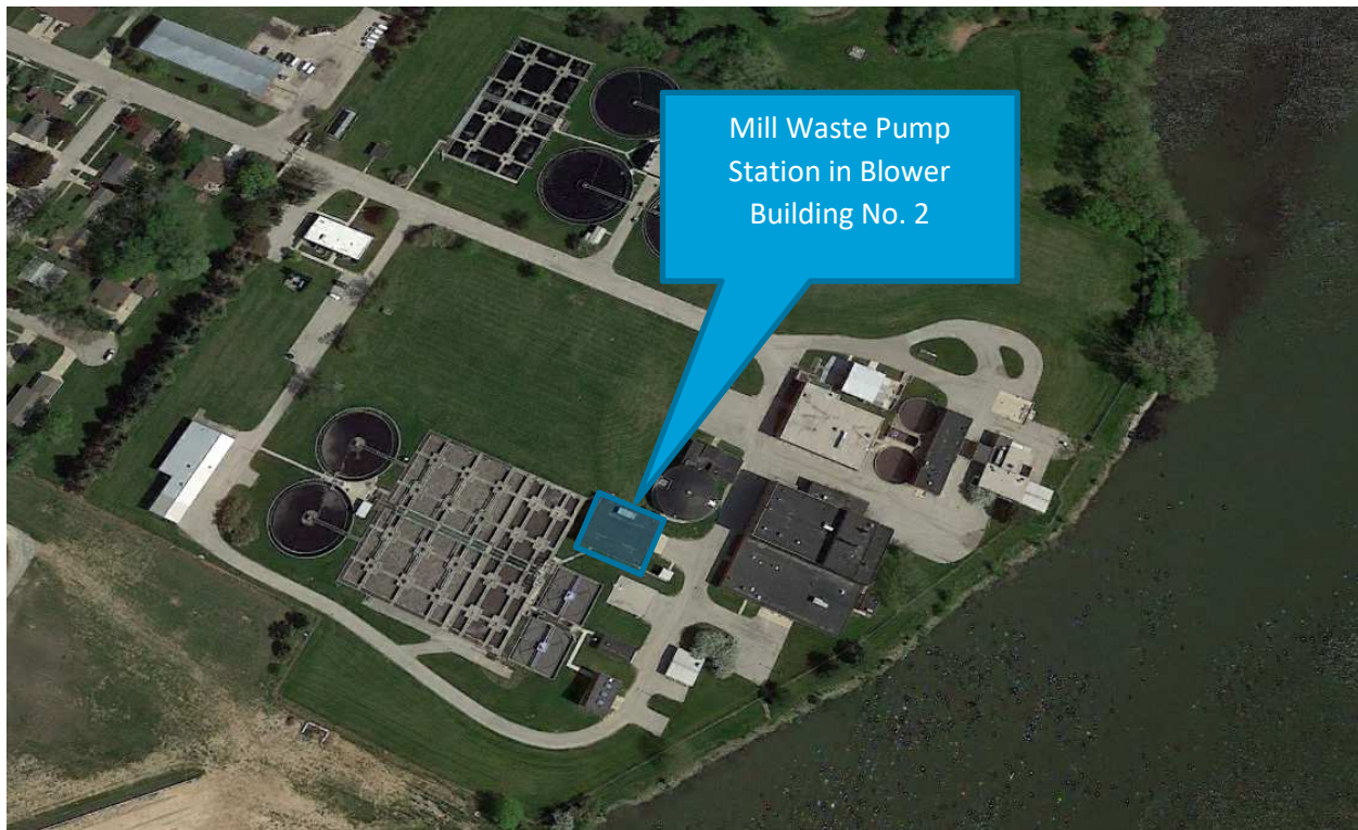
Figure 3-3 Location of Existing DPF Mill Waste Pump Station
