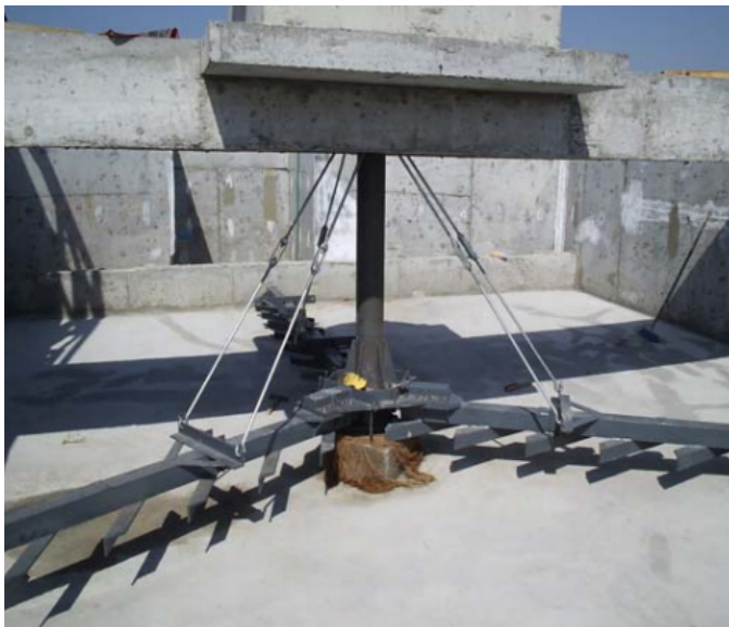
Figure 4-2 Detritor Tank Interior ( Limited, 2009 )
