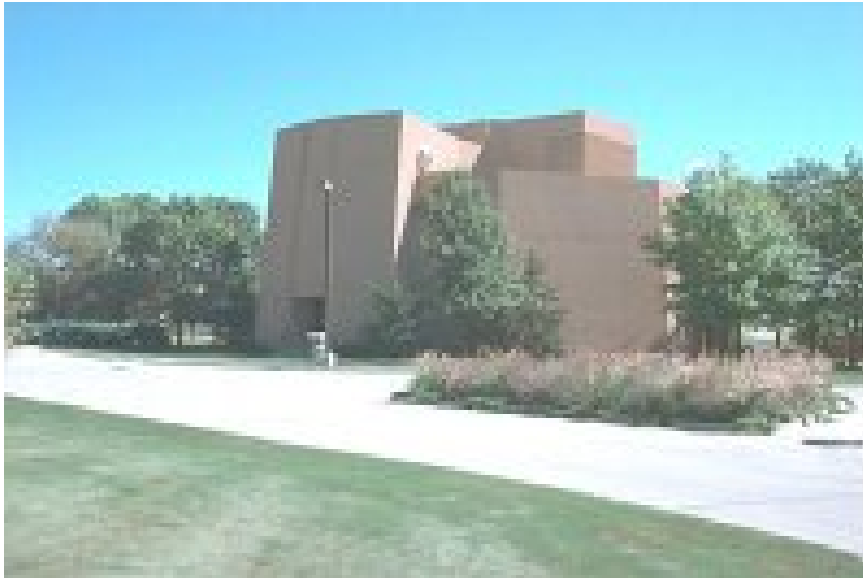
Figure 3-2 Influent Pump Station
