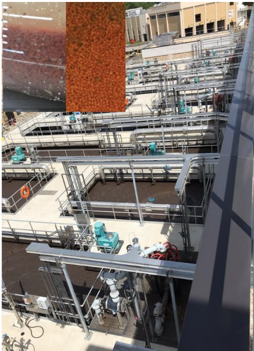
Figure 5-4 Image of the DC Water DEMON System with Inset Anammox Granules (Images Courtesy of DC Water)
