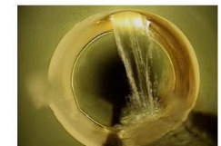
Picture above: Likely illicit sump pump connection discharging inflow of clear water into sanitary sewer. NEW Water Television Program 9/5/2018
